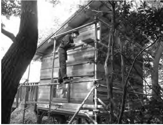
Figure 16. Making the walls of the house (2010)
