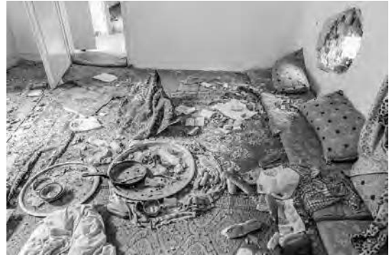
Figure 9. This was the saddest moment I personally experienced, which was surely not sadder and more brutal than what some civilian residents of Sur district suffered; loss of homes, injuries, even death... The large hole on the wall in the right-hand side is a puncture caused by a loose artillery shell, that instantly killed an old woman having a meal at her home, away from the conflict area. The place was left as was and nobody has cleared the scene, including the relatives of the old woman. ©Murat Germen, 2016.
