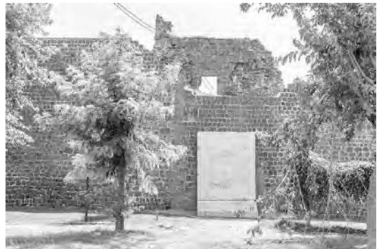
Figure 6. The various entrances, gates through the old city wall that were previously accessible to public, are all sealed off now with huge concrete blocks for security purposes. ©Murat Germen, 2016.
