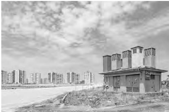
Figure 4. The new housing development is not constructed in a way compatible with the relatively harsh climatic conditions, which get very hot during the summers and cold in winters. The old Sur district has narrow streets, adjacent houses, thicker stone walls in older buildings and internal courtyards that provide comfortable living environments in all seasons. The new buildings are energy-inefficient and are devoid of regional character since they look the same as buildings anywhere else in Turkey. ©Murat Germen, 2016.
