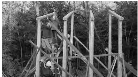
Figure 15. Raising the house beams (2008)
